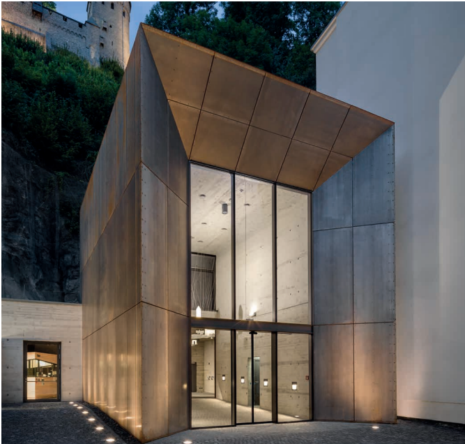
Experience Elevator Castle Altena – Steel façades made of patinax®. Source: AMS GmbH, www.ams-mbt.de
