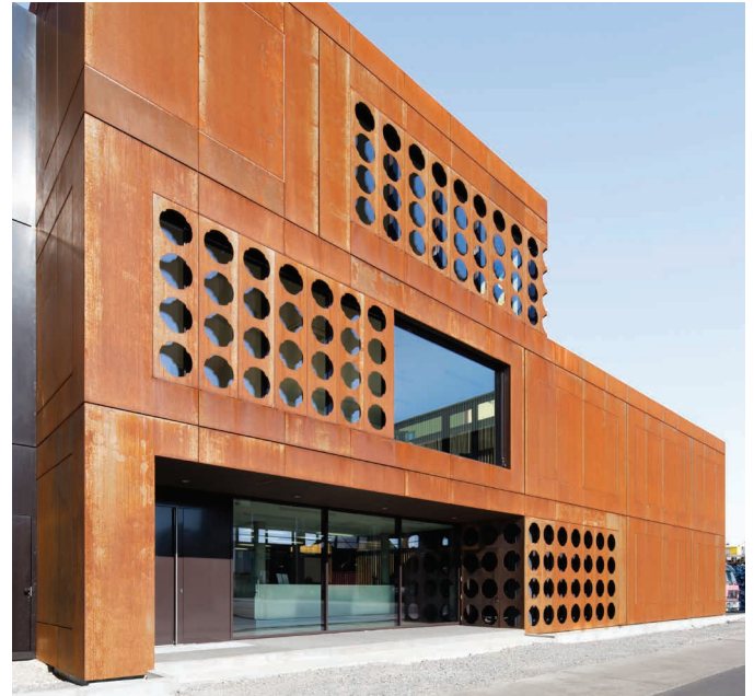
Raw materials trading Georg Lech in Schweinfurt – Steel façades made of patinax®.
