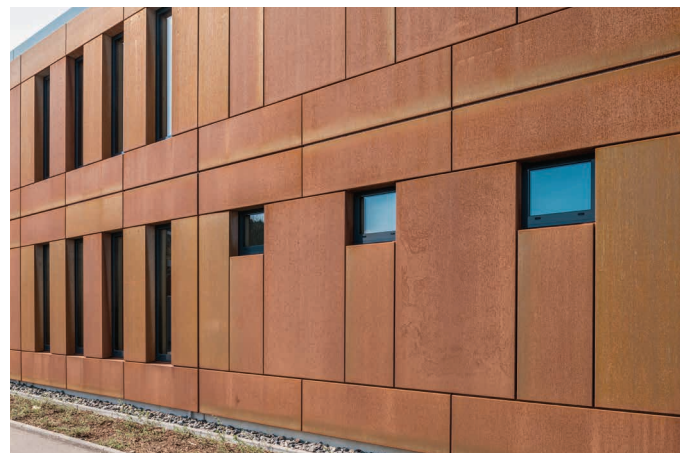
Weathering steel in use – Façades panels made of patinax®. Source: AMS GmbH, www.ams-mbt.de
