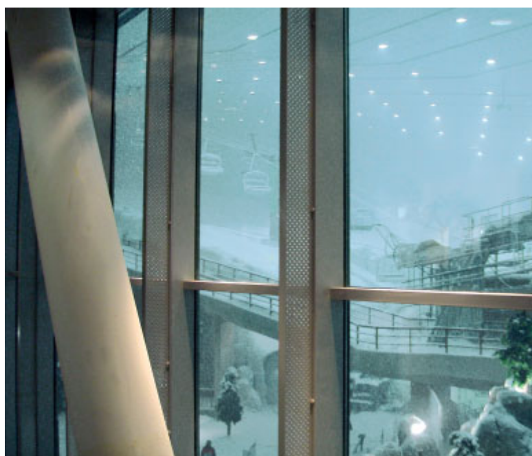
▲ Double-T beams from ThyssenKrupp DAVEX form the backbone of the glass façade between the Dubai indoor skiing center and the adjacent shopping mall. In addition, 5000 curious visitors come to see the structure every day.
