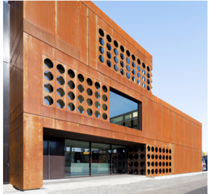
Raw materials trading Georg Lech in Schweinfurt – steel façades made of patinax®.
