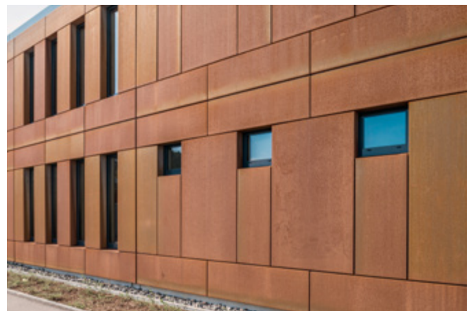
Weathering steel in use – Façades panels made of patinax®. Source: AMS GmbH, www.ams-mbt.de
